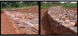
The retaining walls has been constructed followed by garland drain at the toe of the dumps and gabion box of have been
